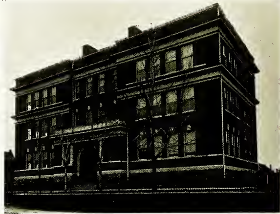
Public School Building, Courtright Avenue
